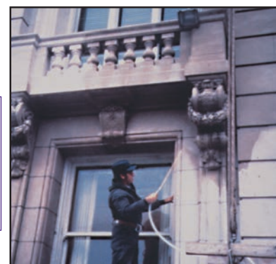
Figure 6. Spray application of silanes on large structures.
